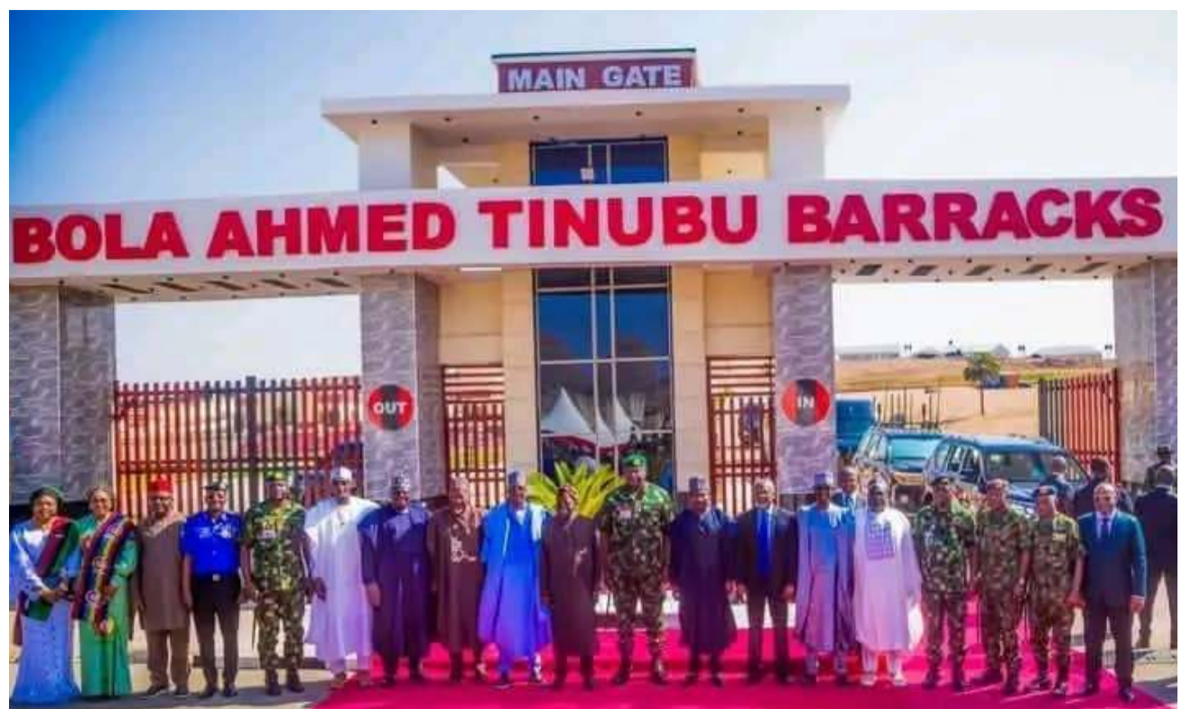
The newly built Bola Ahmed Tinubu Barracks in Abuja, commissioned with the aim of improving the living conditions of dedicated soldiers and their families.
